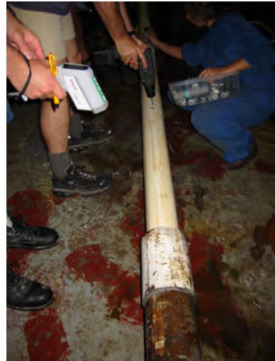
Figure 18. Holes were drilled in the liner at 1-meter intervals to relieve potential gas overpressures, and a digital thermometer was inserted to record internal sediment temperature.
